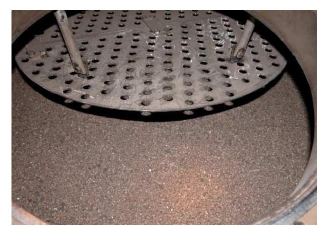
View into Oxi reactor 1320 through manhole Catalyst last changed in 2002 (mist and droplets from process caused deposits and increased pressure drop, that was the reason catalyst had to be changed)
